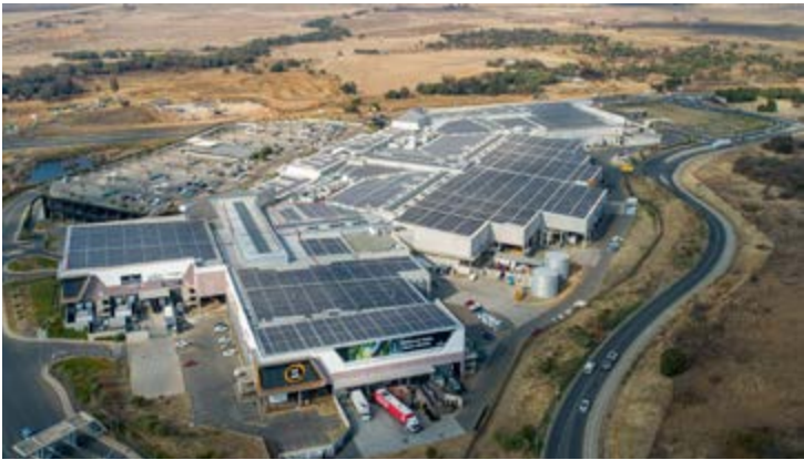
Mall of the South, Johannesburg, one of the top 10 largest solar PV installations
